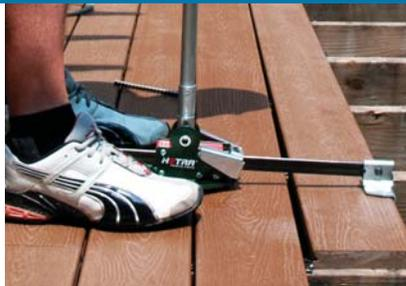
Begin the next board by sliding the board onto the double leg side of the deck clips. Make sure the new deck board is secured tightly against the deck clips for consistent gapping. Repeat steps 2 and 3.
