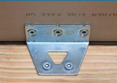
The first deck board needs to be fastened using angle brackets before using the clips. Use Deckmaster Hidden Deck Angle Brackets (HDA), item number DMHDACP. Fasten the HDA bracket to the bottom of the first deck board, then secure it to the header plate. Using the HDA bracket allows the first deck board to be fastened without screwing down through the top. Use Deckmaster clips once the first board has been installed.
