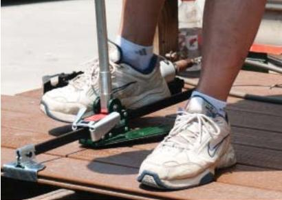
Repeat steps 2, 3 and 4 until the last deck board. Repeat step 1 to install the last deck board using the Deckmaster Hidden Deck Angel brackets.
