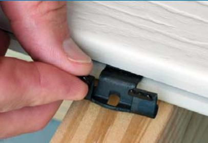
Insert Deckmaster clips into the groove in the deck board at each joist.
