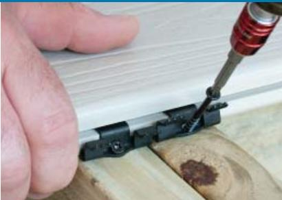
Butt joints should be attached using two deck clips for additional strength. Using two clips at butt joints will allow for any shrinkage, swelling or other movement that may occur. The second clip may be added by scabbing a runner board to the joist and attaching a deck clip.
